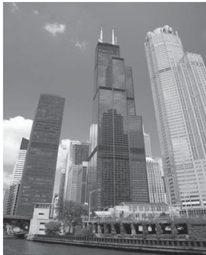
(b) The 110-stories high, 442-m tall Willis Tower (formerly known as Sears Tower), in Chicago, Illinois, USA. Designed by architects, Skidmore, Owings, and Merrill and structural engineer Fazlur Khan, and completed in 1973, it is the tallest building in the western hemisphere. The superstructure consisting of nine interlocking rigid steel framed tubes that terminate at different heights, efficiently counteract all lateral and gravity loads.
