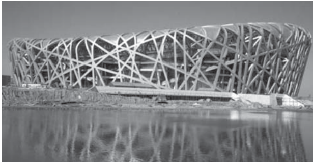
(c) Beijing National Stadium, also known as Bird's Nest, built for 2008 Summer Olympics in Beijing, China, and is the world's largest steel structure. This 91,000-seat stadium was designed by Swiss architects Herzog and de Meuron, ArupSport, and China Architectural Design & Research Group. It is 330-m long, 220-m wide, 69.2-m tall and contains 110,000 tonnes of steel.
