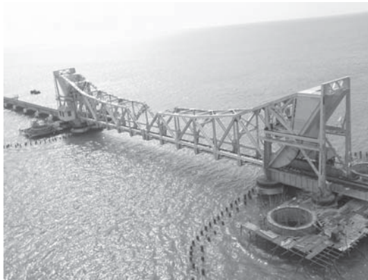
(a) The 2,065-m long Pamban railway bridge, on the Palk Strait, connects Rameswaram to mainland India. Constructed in 1914, it is still in good condition and considered as one of the marvels of engineering. The double-leaf bascule bridge section shown in this picture can be raised to let ships pass under the bridge. The bridge is located at the world's second highly corrosive environment (next to Miami, US), which is also a cyclone-prone, high wind velocity zone.
