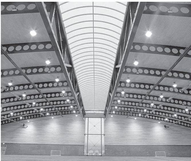
Fig. 1.12 Cellular beams over Rangers FC, an indoor training facility in Scotland (Courtesy: ASD Westok Ltd, UK)
