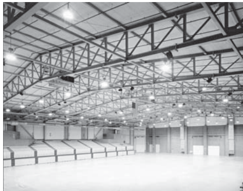
(d) A typical pre-engineered building for the American Royal Exhibition Hall and Arena, Kansas City, MO. They are adopted for low-rise buildings with an eave height of up to 30 m and can be very economical and speedy. (Photo: www.butlermfg.com )
