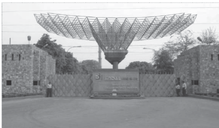
Fig. 1.13 Stainless steel double-layer grid roof at Hissar, Haryana
