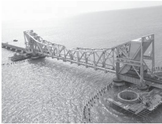
(a) The 2,065-m long Pamban railway bridge, on the Palk Strait, connects Rameswaram to mainland India. Constructed in 1914, it is still in good condition and considered as one of the marvels of engineering. The double-leaf bascule bridge section shown in this picture can be raised to let ships pass under the bridge. The bridge is located at the world's second highly corrosive environment (next to Miami, US), which is also a cyclone-prone, high wind velocity zone.
